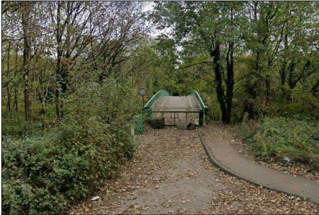
Figure 18: Existing bridge crossing PRoW across A48
